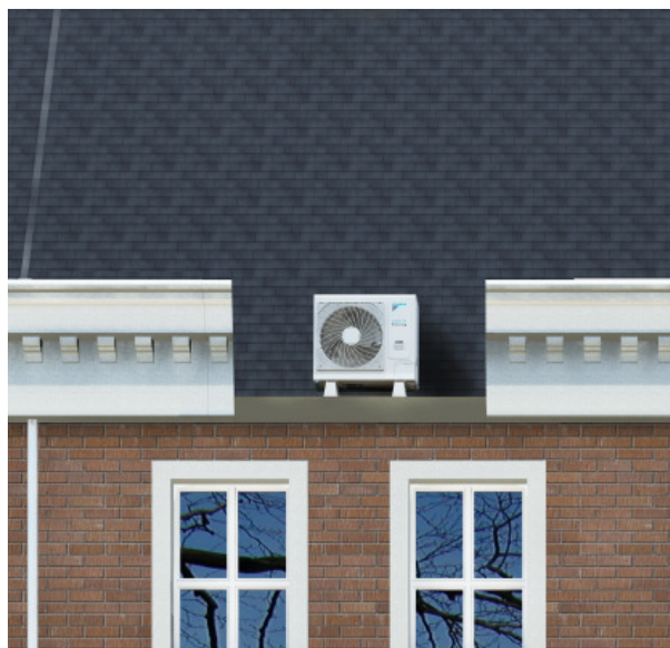
Example of VRV-S series behind a parapet
