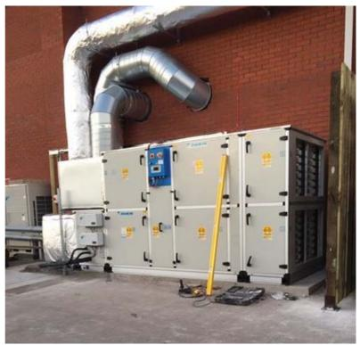
The AHU and condensing units are in a service area at the rear of the building, and enclosed by a wooden fence for neatness and security.
