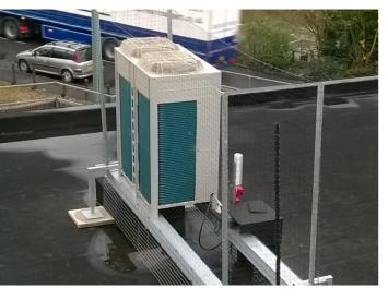
The Daikin Altherma Flex units were installed in a decentralised configuration by Daikin installer Moore of Devizes. Director Les Moore says: "The heat pump condensing units are on a new steel platform on the roof, with hydrobox units and matching hot water cylinders in each flat."
