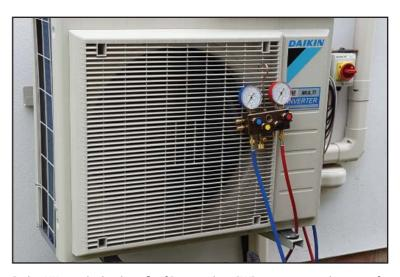
Daikin UK says the key benefit of R32 is its low GWP – 675 against the 2088 of R410a – which makes it an ideal refrigerant to use through the phase-down of HFC gases. Used on its own, R32 is actually more efficient than R410a, and this leads to other benefits such as systems requiring a smaller refrigerant charge.
