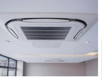
The systems include Seasonal Classic and Active models from the Sky Air range and a single multi-split. Indoors, the cooling or heating is delivered by 13 Roundflow cassettes of 5kW or 7.1kW and five wall-mounted inverter units of 2.5kW or 3.5kW.
