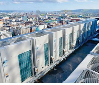
In addition to the heat recovery units, the podium plant area has three Daikin VRV IV heat pumps serving DX coils in the hotel's air handling units. It also has the outdoor units for Split and Sky Air systems that provide cooling for the laundry and communications room.
