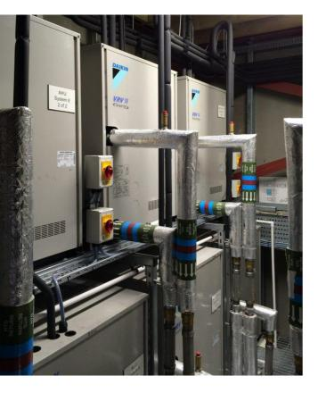
Six systems totalling 13 condensers generate the total heating and cooling requirement for all floors and an air curtain in the lobby. Another four condensers serve the building's two air handling units, which supply tempered air at 18oC to the rear of fan coil units (FCUs) throughout the building. The building's total calculated load is 427kW (peak instantaneous: 348kW).
