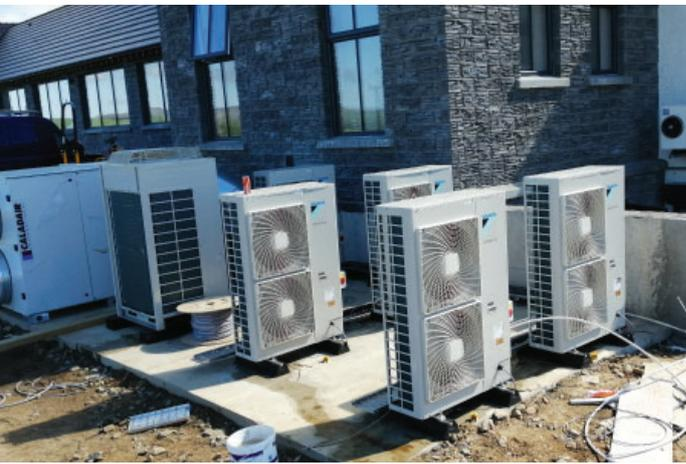
The three-phase Daikin Altherma HT heat pumps installed at the Salhouse deliver water at 80°C without electrical heating. This is achieved through a two-stage compression process: there are R410A refrigerant circuits in the outdoor units and R134A circuits in the corresponding indoor units.
