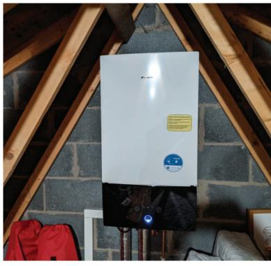
Richard McLaren says: "The wall-mounted indoor unit, which contains the controls and hydraulic components for the heating system, is installed in the attic above the utility room. The indoor temperature controller is in the hallway.
