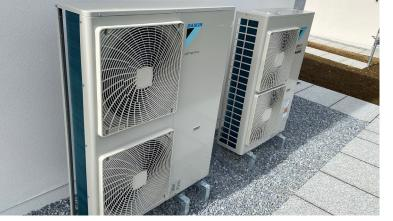
A new gas injection scroll compressor ensures reliable performance in sub-zero outdoor temperatures and supports a 35% improvement in heating capacity. A leaving water temperature of 60°C can be achieved, even when it is -10°C outdoors.
